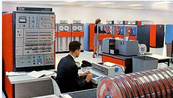
Typical "mainframe" computer: IBM 360/50
